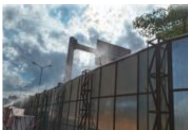
Wall block automatic spray system
